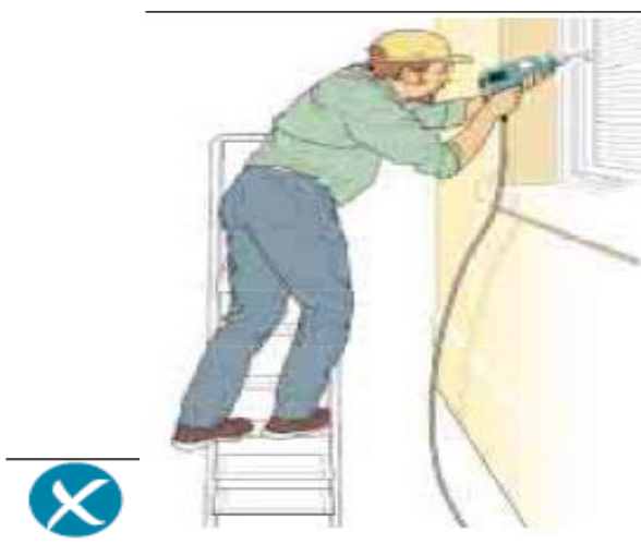
Incorrect – steps side on to work activity
