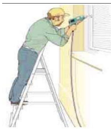
Correct – steps facing work activity
